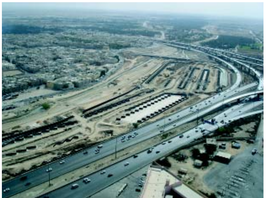
Bioremediation Facility Under construction
