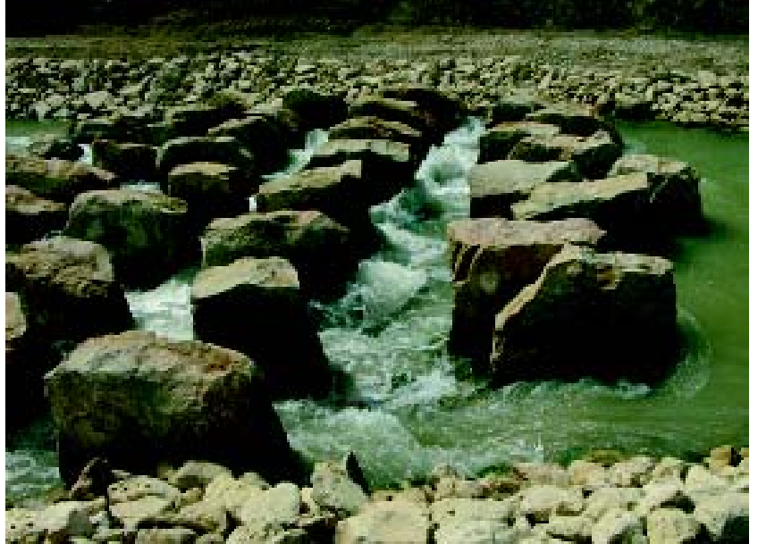
Typical Natural Stone Weir in the Dry Weather Flow Channel
